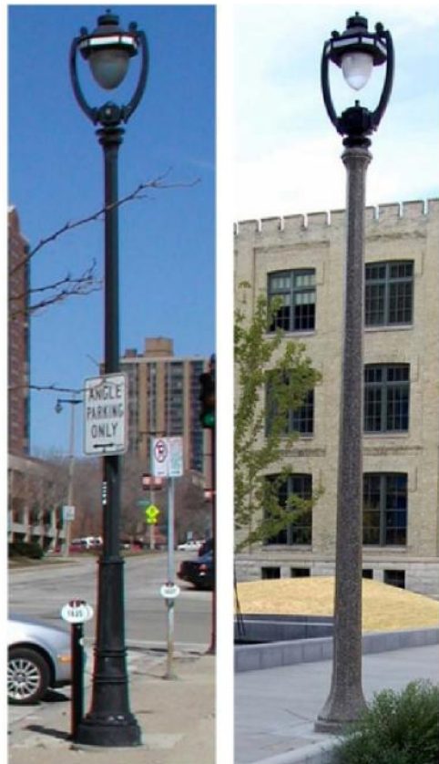
Typical pedestrian-level Milwaukee Harp Lamps 32
