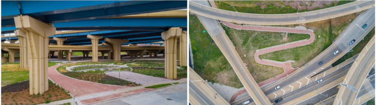
The green Infrastructure plaza and path located under the Marquette Interchange 48
