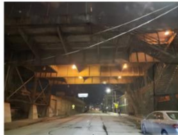
Underpass N 16thSt Viaduct
